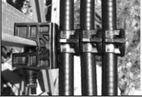
Maximum loading: 3 polymer hangers (shown) or two metal hangers.
