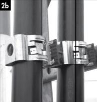
Snap hanger into isolator (2a). Always alternate hanger and isolator to prevent loose metal-tometal contact.
