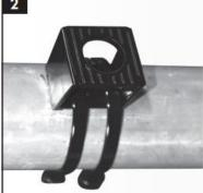
Tighten the snap-in hanger adapter to the round tower member with two nylon cable ties or two wraps of outdoor rated cable banding. Cut off and discard remaining tail.
