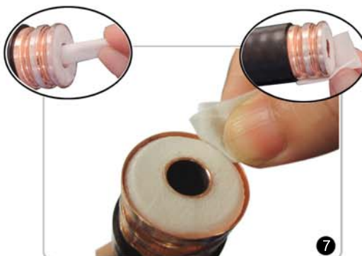
Open up the alcohol pad to clean the inner side of center conductor, the insulator and outer corrugation carefully as per picture shown.
